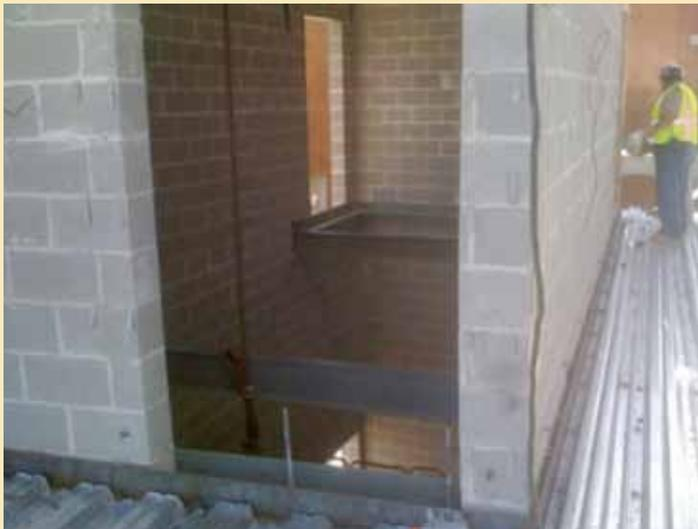
to accept the safety cables. The guarding of interior floor opening by planking, plywood, or other methods is also typically addressed by the steel erection during the bidding process. Unfortunately, potential fall hazards at stairway and elevator shaft openings continue to exist, and the responsibility to provide common guarding or barricades has often been overlooked.
